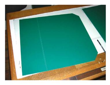
5. Cut out the top. The top is 20 3/8" by 15.5" with the grain running the 20 3/8" direction (same as the bottom/back side). If faced with a rib of the Coroplast, lean toward having the top a little shorter in the 15.5" dimension.
